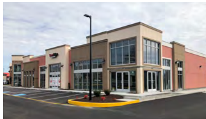
Completed 1305 S. Salisbury Blvd.
